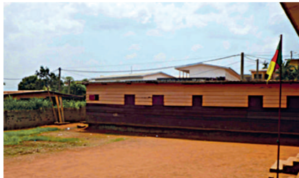
Ferrero Social Enterprise In Cameroon. Cité Verte Kindergarten Project: current wooden building
